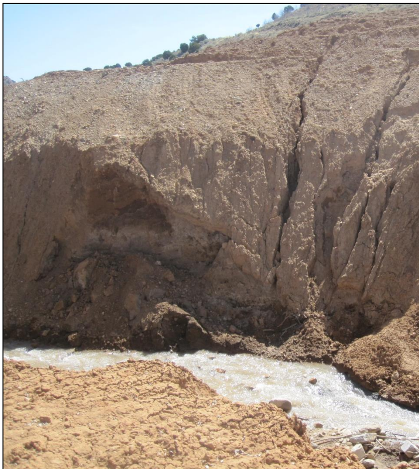
Figure 5.9. Streambank erosion occurring in the South Fork Chalk Creek subwatershed.
